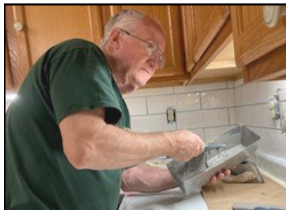
Dave Lindley grouting the newly installed kitchen tile.
